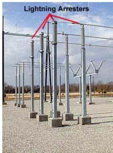
Fig(1)-Lighting arrester on bus structures
